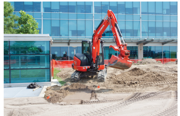
Greenhorizons' Ultimate Sports Turf System™ installation.
