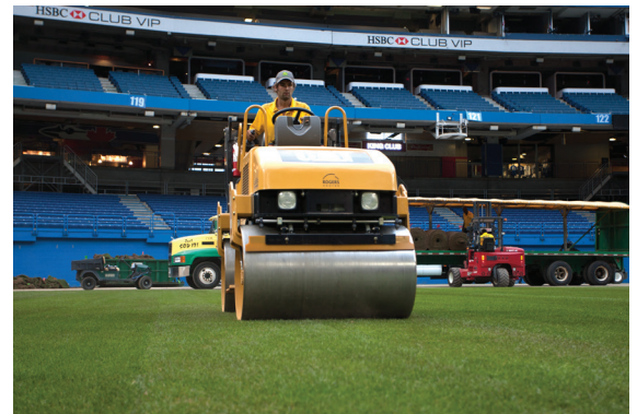
Rolling the field to ensure it was firmly adhered to the concrete floor.
